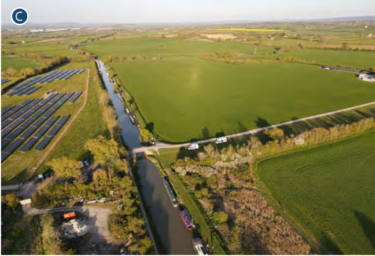
The topography rises gently from the canal toward the south east.
